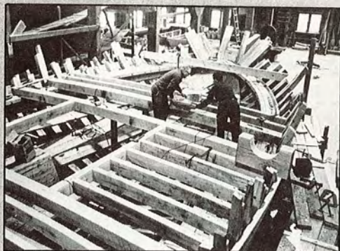
Work in progress . . . the sloop under construction at Harvey Gamage Shipyards, winter, 1969
