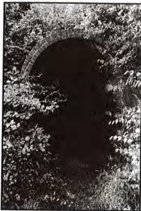
One of the Point's still-functioning brick caves
